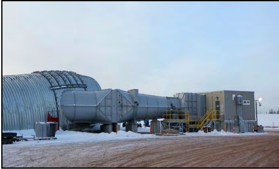
Portal heater house and ducting, Dec. 2013
