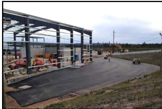
Paving applied to re-seal contact area, November 2013
