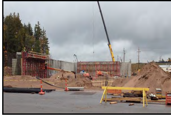
COSA concrete foundation & sidewalls, October 2013
