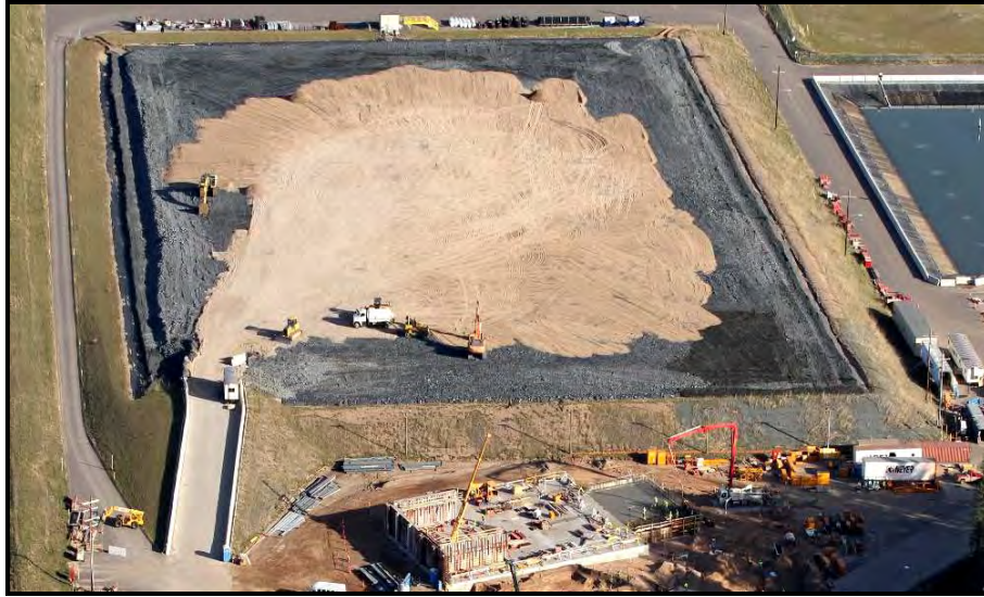
Limestone being applied to TDRSA in preparation of covering, October 2013
