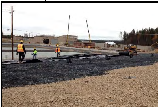
Rolling out the geo-membrane for cover, Oct. 2013
