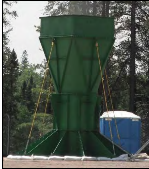
Temporary air ventilation exhaust fan, June 2013
