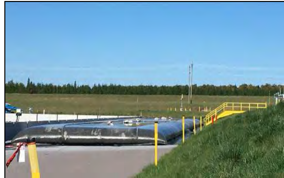
Geotubes dewatering west of CWB 2, September 2016
