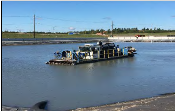
Dredge performing sediment removal, September 2016
