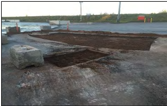
Removal of worn asphalt prior to repair, September
