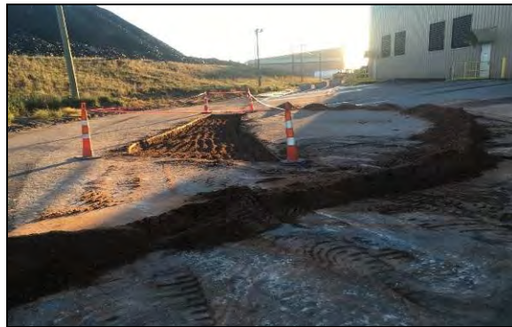
Removal of worn asphalt prior to repair, September 2016
