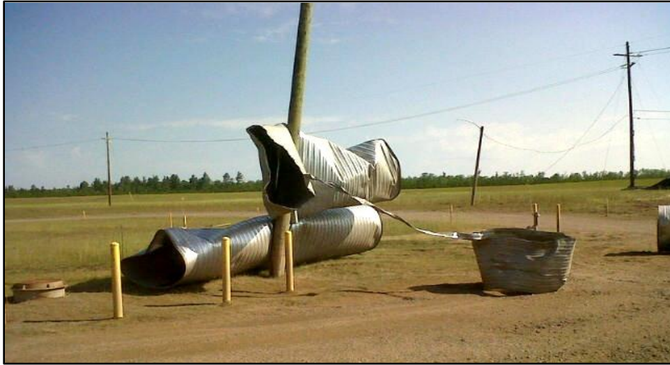
Vent Tube Wrapped Around Light Pole
