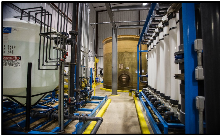
Water Treatment Plant Ultrafiltration Units, August 2015
