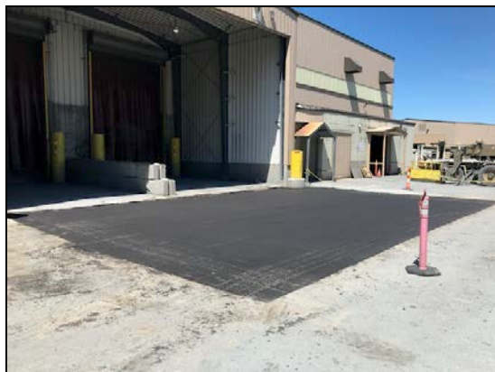
COSA Repairs Made to Worn Asphalt, June 2019
