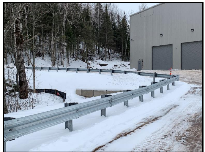
Left: Erosion on access road corner, July 2020. Right: Retaining Wall, Silt Fence, and Guard Rail Additions and Improvements at the WTP Loading Dock, December 2020.
