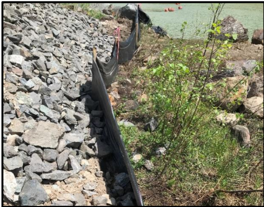
Maintained silt fence on the South side of the HTDF during construction activities, Summer 2020
