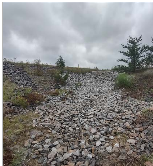
NCWIB #3 – After riprap repairs
