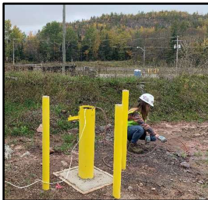
Left: Development of one of the newly installed wells, September 2021. Right: Auto-Profiler purchased and installed in 2018.
