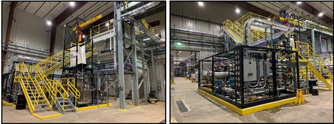
Left: Remineralization System, May 2021. Right: Concentrator RO, May 2021
