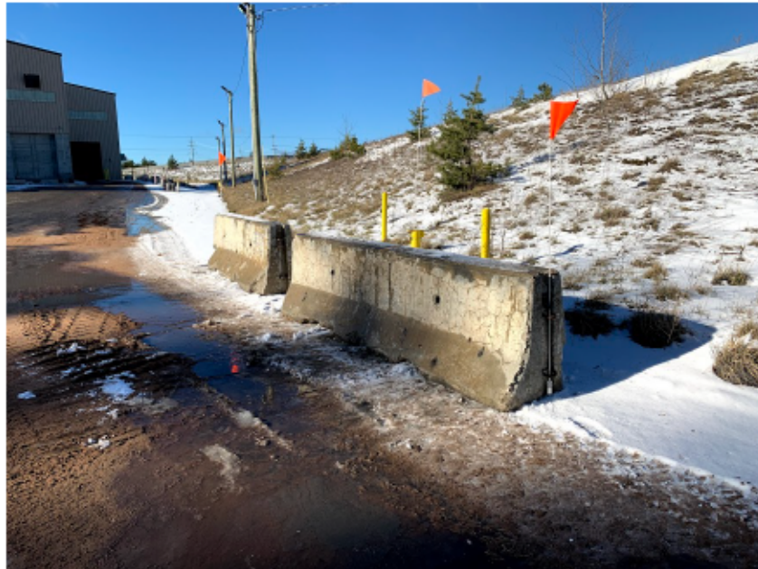
Barriers installed near QAL067A; December 2020
