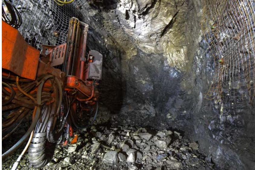
Bolter installing ground support in Eagle East heading
